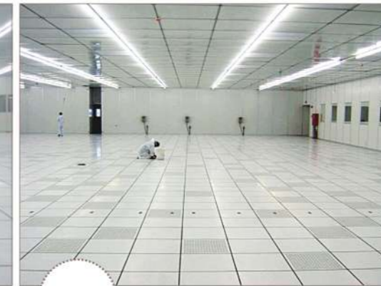
10K级净化房 10K class clean room
